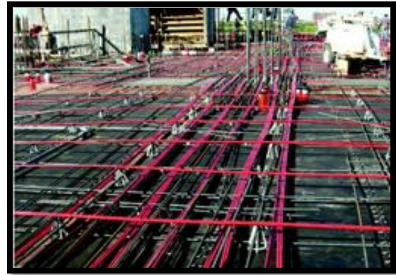
Two-Way Post Tension before pour concrete
